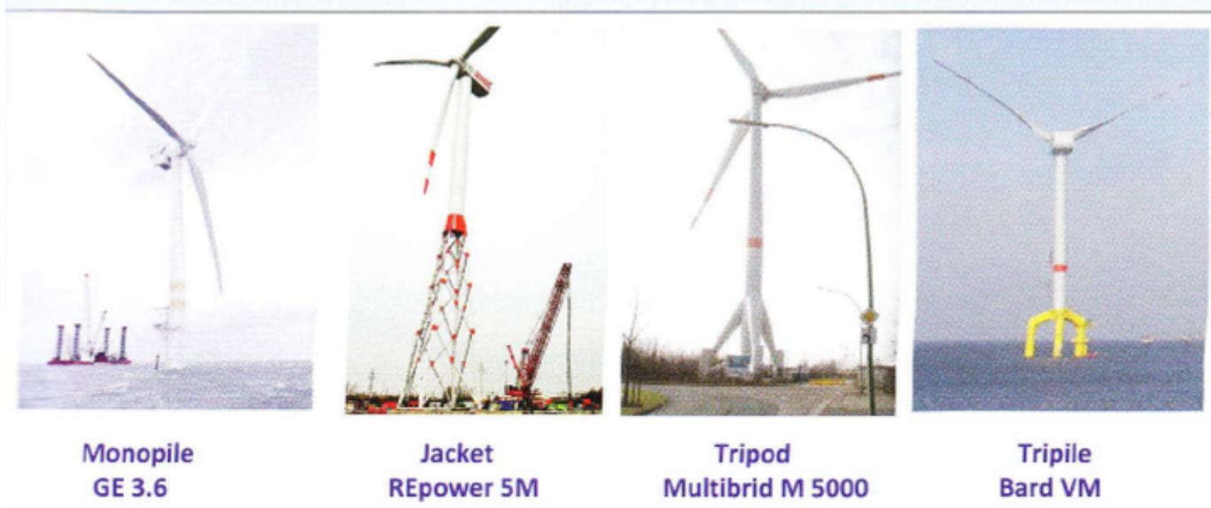
**Fig. 13:** Four different offshore foundation designs for wind turbines of the multi-megawatt size
