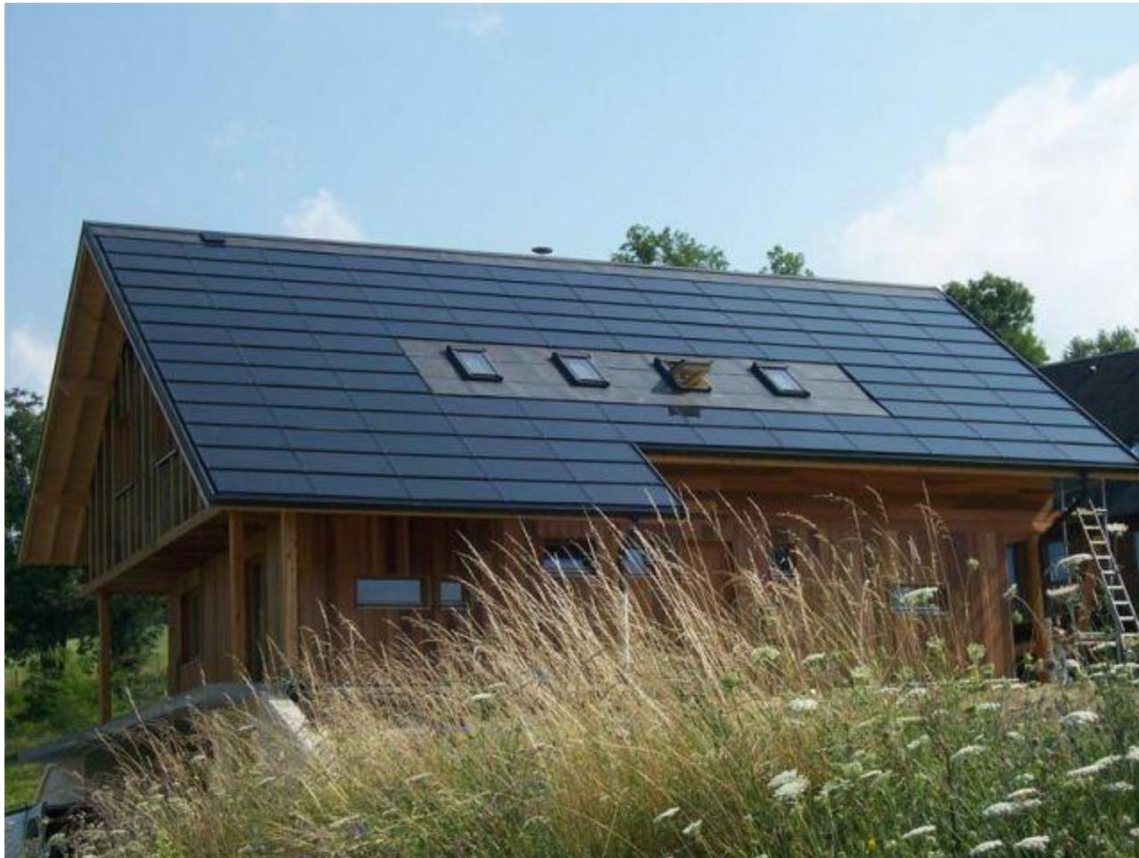
PV System CIS (Sulfurcell) 13.5 kWp 12 000 kWh/year
